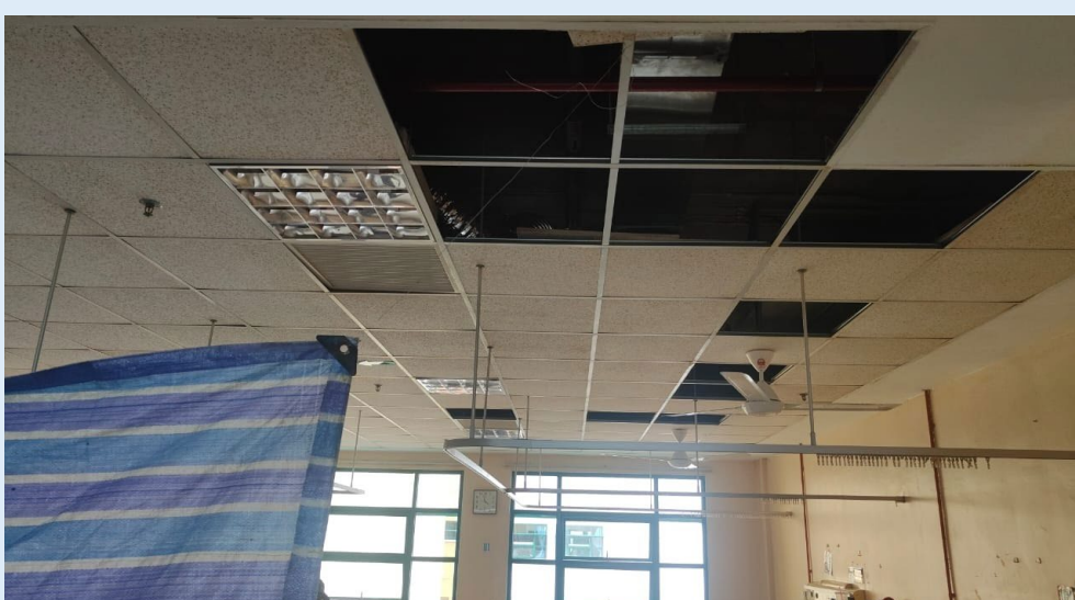
Ceiling clearance to install air-conditioners
