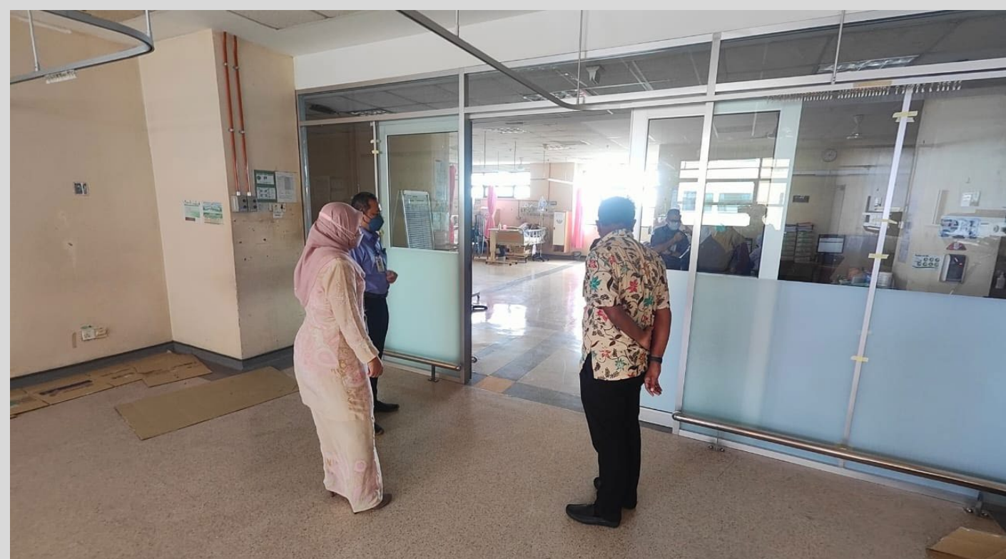
Site visit by hospital admin and engineer
